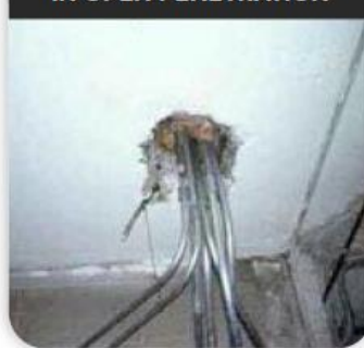
NO FIRE STOPPING IN OPEN PENETRATION
